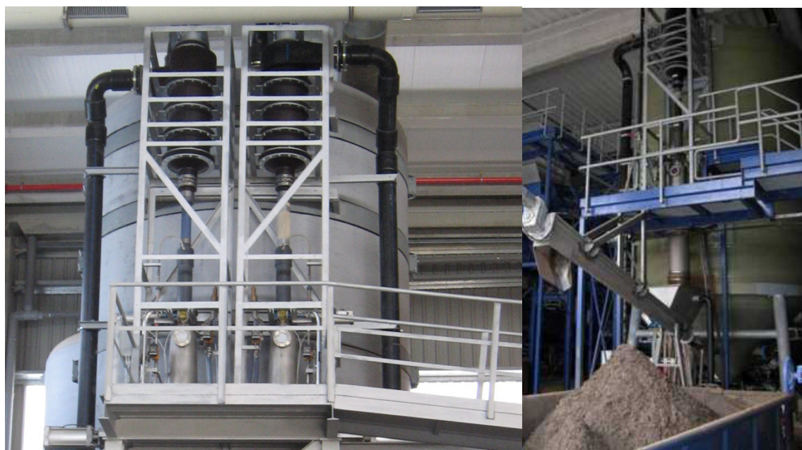
Fig. 4.6: a) Grit Removal System at Granollers, Spain b) Grit classifier at Mühlheim, Germany
