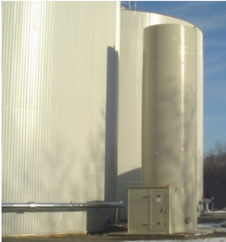
Fig. 4.14: External Biological desulphurization
