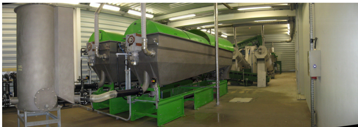
Fig. 4.10: Thickener units in Valorlis, Portugal
