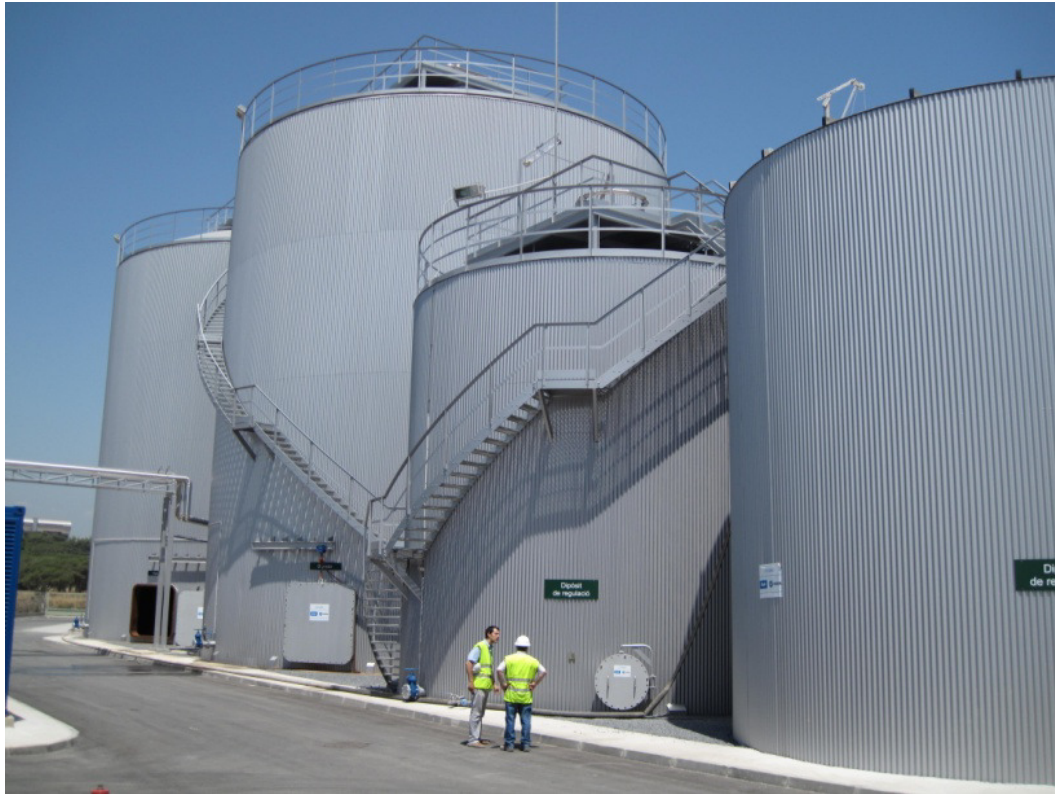
Fig. 4.12: Suspension buffer and anaerobic digester in Granollers, Spain
