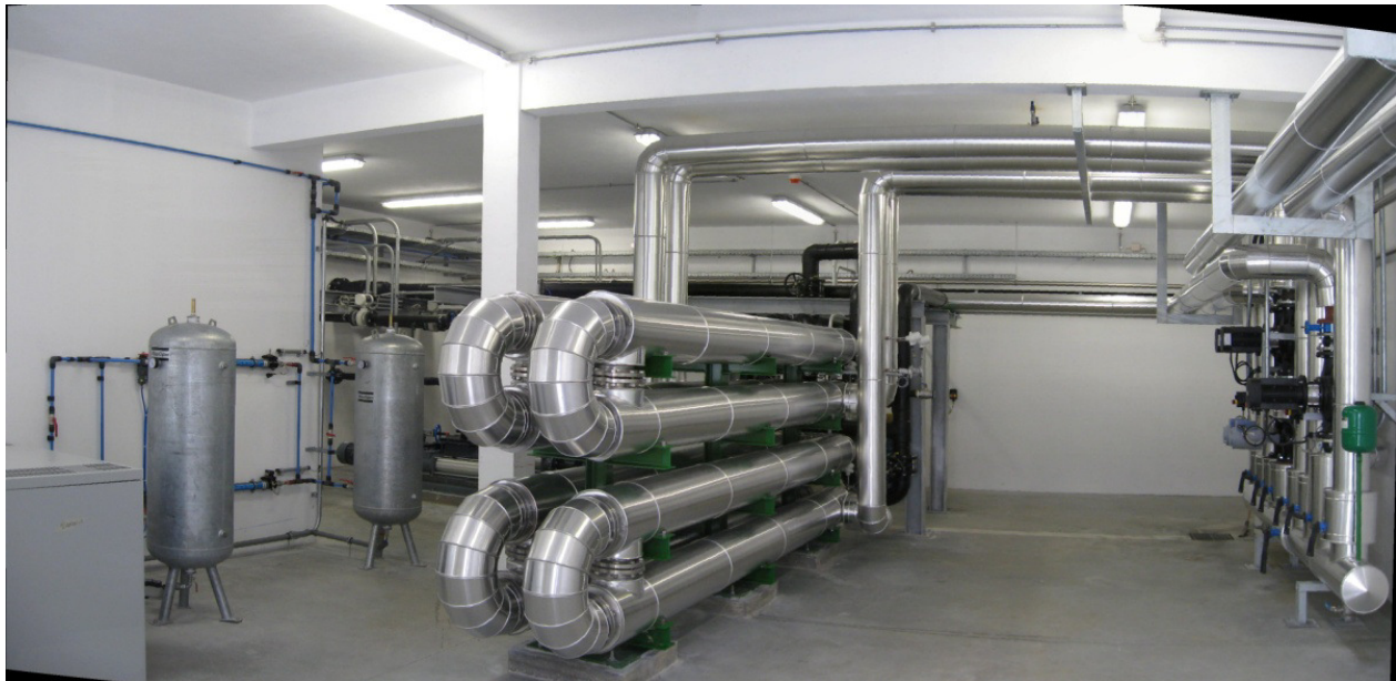
Fig. 4.14: External heat exchangers, Valorlis, Portugal
